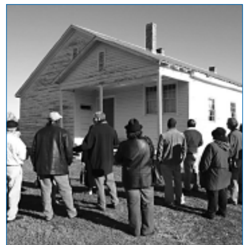
Many historically important schools, such as this former Rosenwald school in North Carolina, can be renovated to serve a community use. Photo by Denise Alexander.
